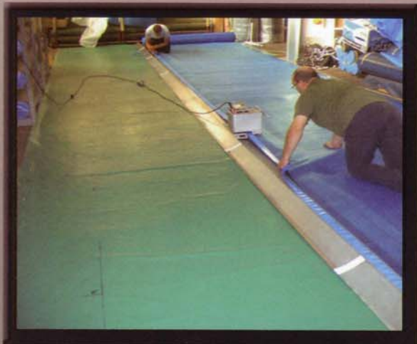
WELDING PE EDGE STRIP TO POOL COVER MATERIAL ITALY
